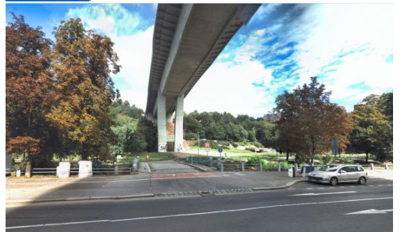
Location E , view from S
