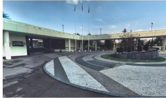
Location B Lower level, view from SE
