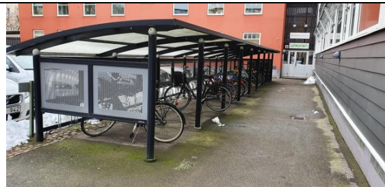
You cannot pass through the object → shall be mapped as a building.
