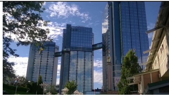
Bridges between buildings are placed too high → shall be omitted.
